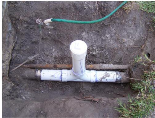
*Figure 4. Sewer Clean-Out and Service Line*
