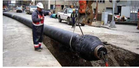
*Figure 2. Pipe Burst Replacement*
