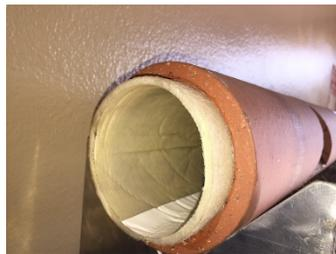
*Figure 5. Cured-In-Place Pipe*
