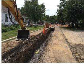
*Figure 1. Open Cut Pipe Replacement*
