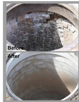
*Figure 6. Lined manhole*
